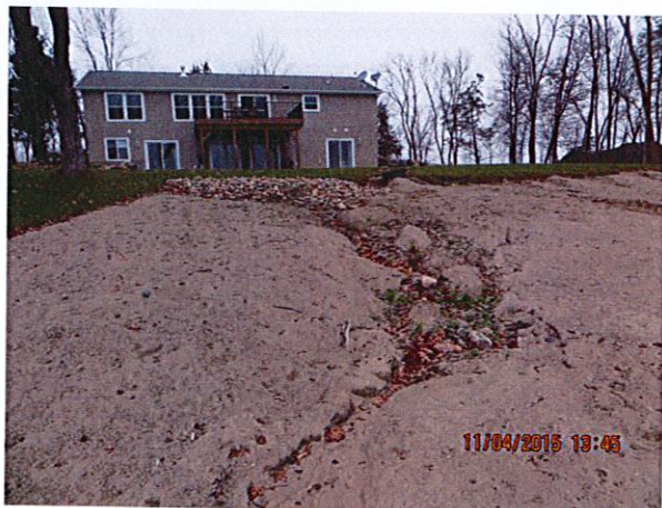
Beach Erosion on Center Lot, looking West
