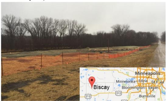
The City of Biscay in McLeod County has a new MSTS (Midsized Soil Treatment System) which replaced 29 of the 51 septic systems in the city. Of the 29 septic systems that were replaced, 21 had been deemed as posing an imminent threat to health. The new system, installed in 2014, is designed for 9,500 gallons per day.
