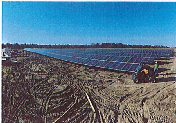
EXAMPLE OF A SOLAR PROJECT IN CONSTRUCTION
