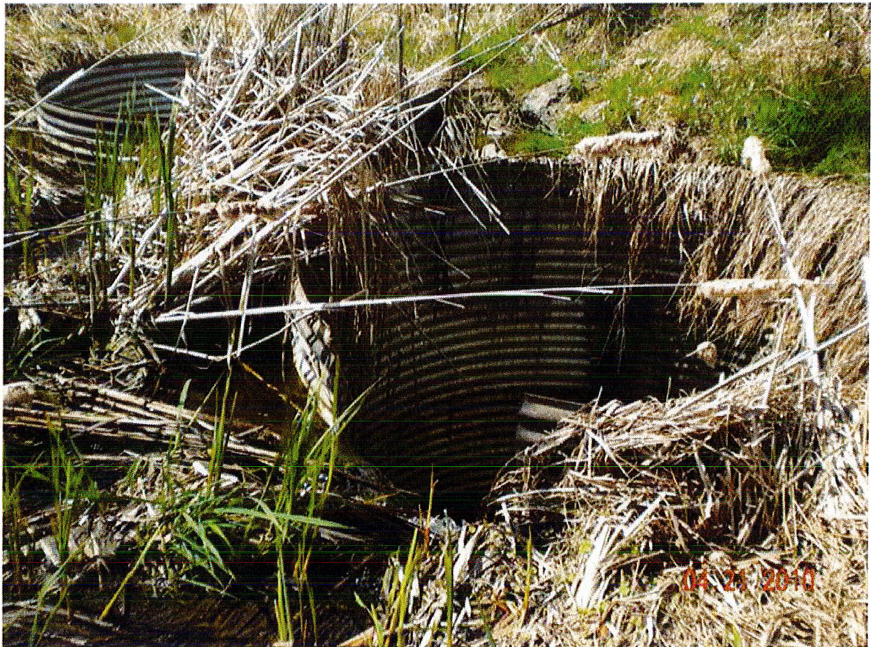
Figure 5: Existing Water Control Structure with Modified North Riser (2010 photo).
