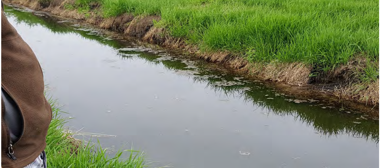
Sloughing from undercutting.
