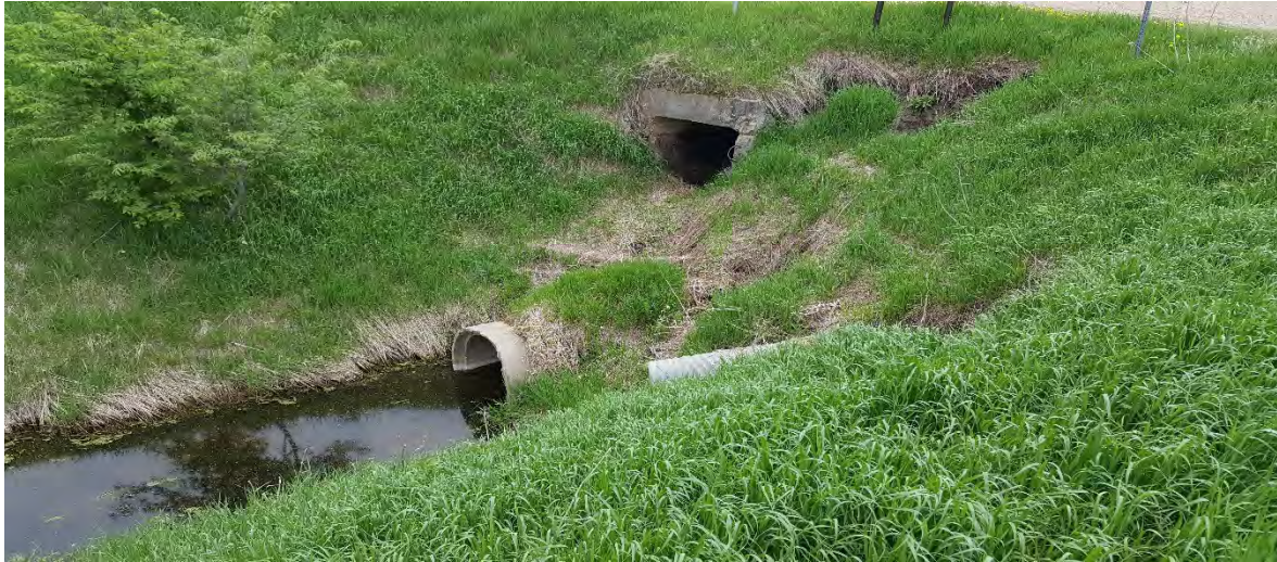
North side of 370 th st. Cement culvert
