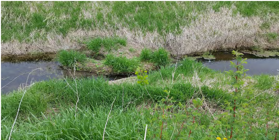
Obstruction in ditch holding about a foot of water back.
