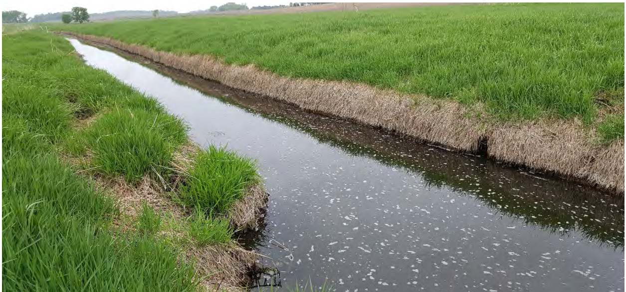
A view of the ditch that was cleaned during the winter, banks have 1:1 slope.
