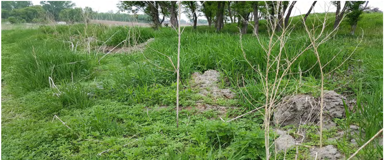
Can see the clay in the un-spread spoils form 2015-2016 winters, the clay would represent digging deeper than the original ditch profile.
