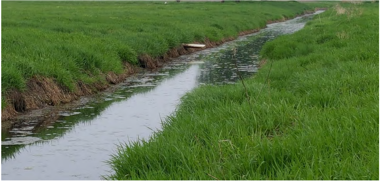
A look at field tile out letting into the ditch. The whole ditch looks like this.
