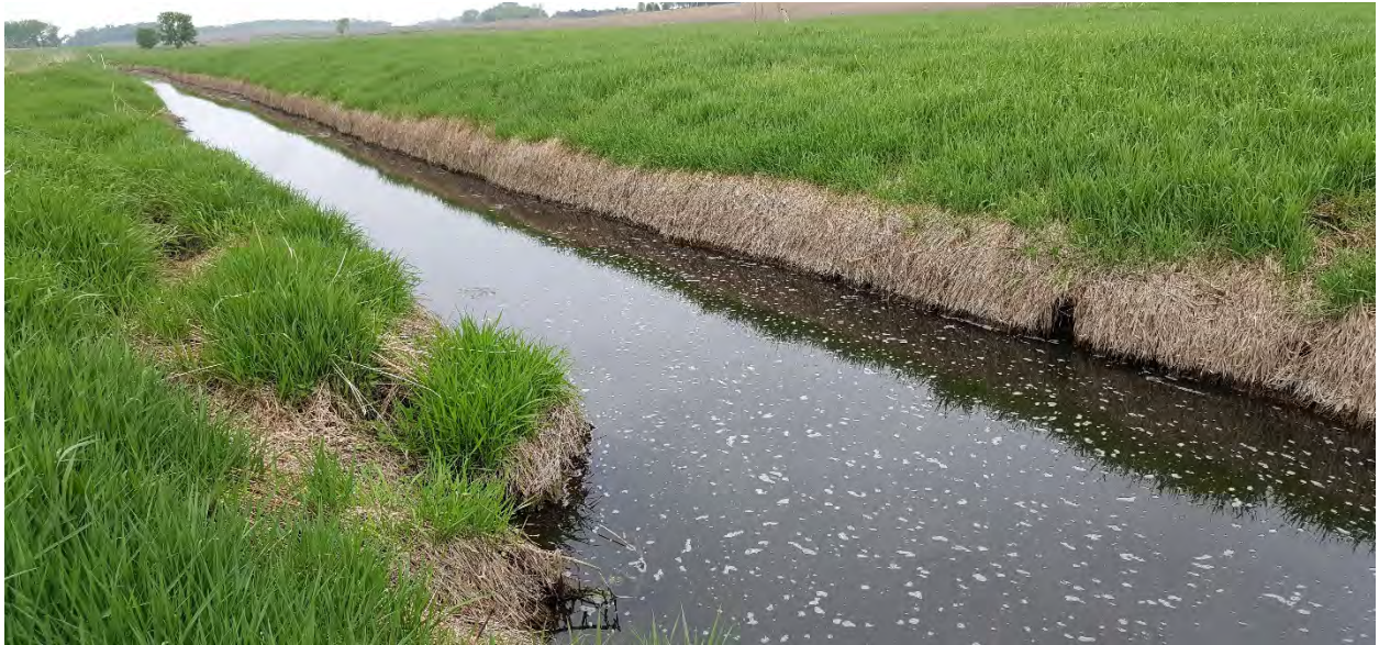
A view of the ditch that was cleaned during the winter, banks have 1:1 slope.
