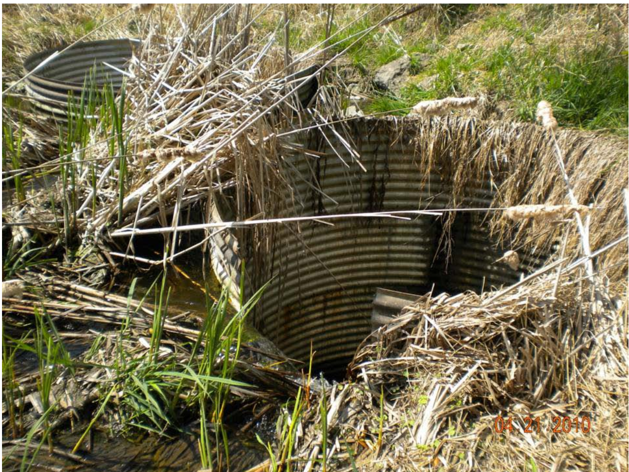
Figure 1. Existing Water Control Structure with Modified North Riser
