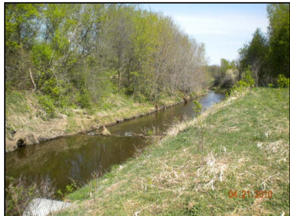
Figure 5. County Ditch 54 Downstream of 96" Risers
