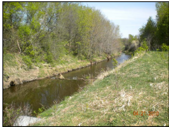
Figure 5. County Ditch 54 Downstream of 96" Risers
