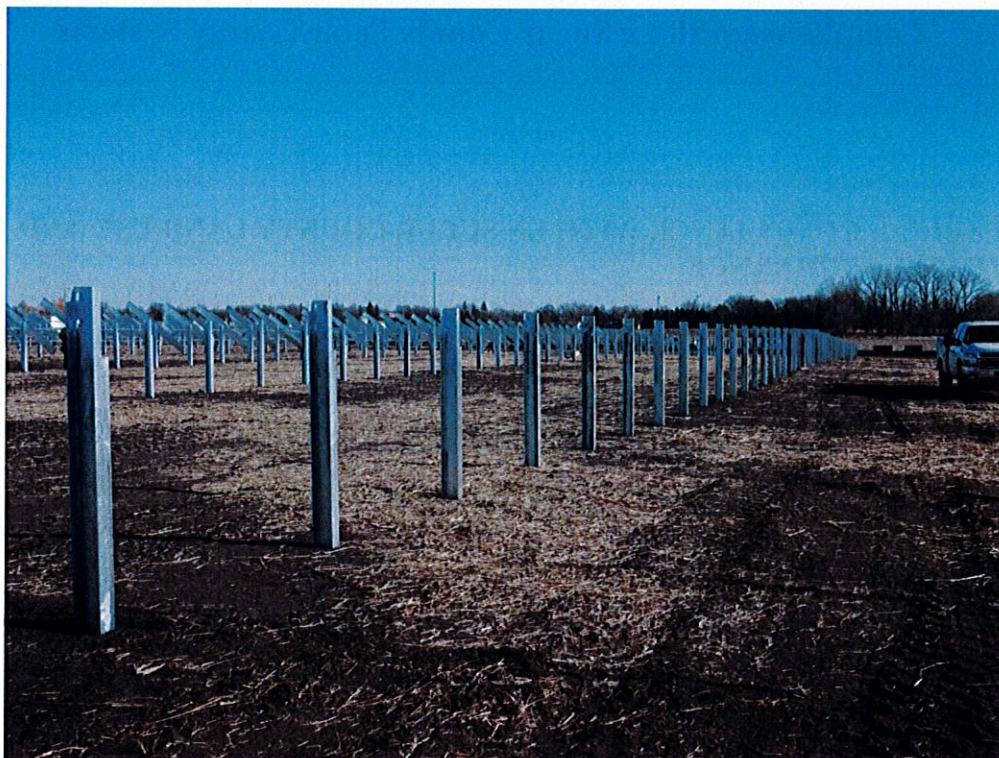
Image 5 – Standard Steel Pier Foundations
