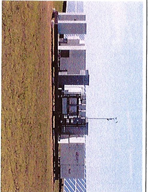
Detail of Switchgear Pad Inverters, Combiner (Junction) boxes, Disconnects Weather Station, Metering
