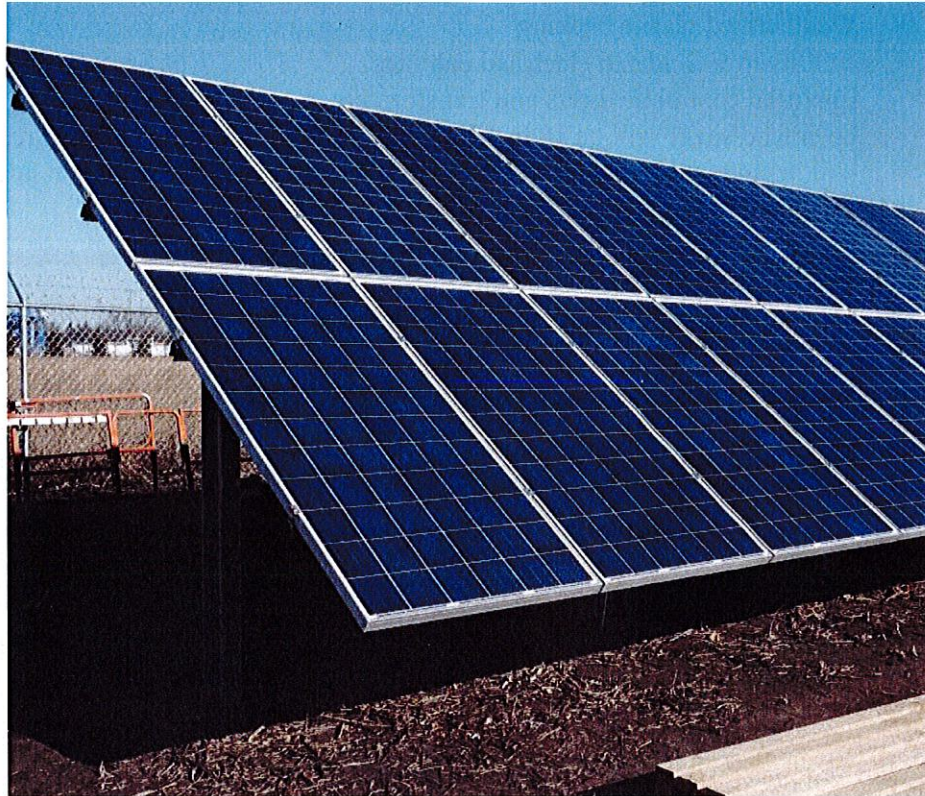
Image 1- Fixed-Tilt System Racking
