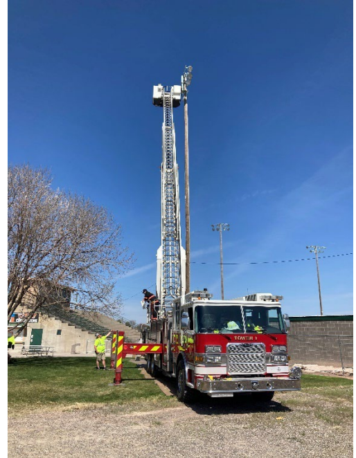
Repairing lights at Cleveland Field
