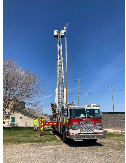
Repairing lights at Cleveland Field
