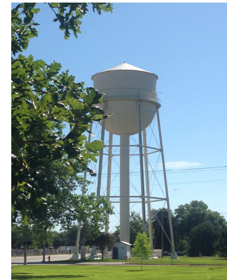
Water Tower - 27th Street & 2nd Avenue
