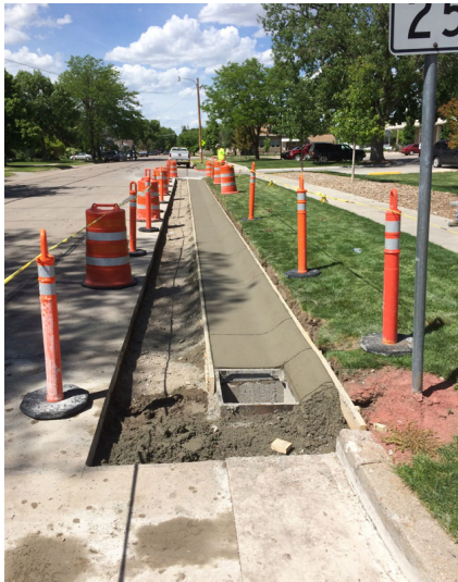
18th Street & 3rd Avenue
