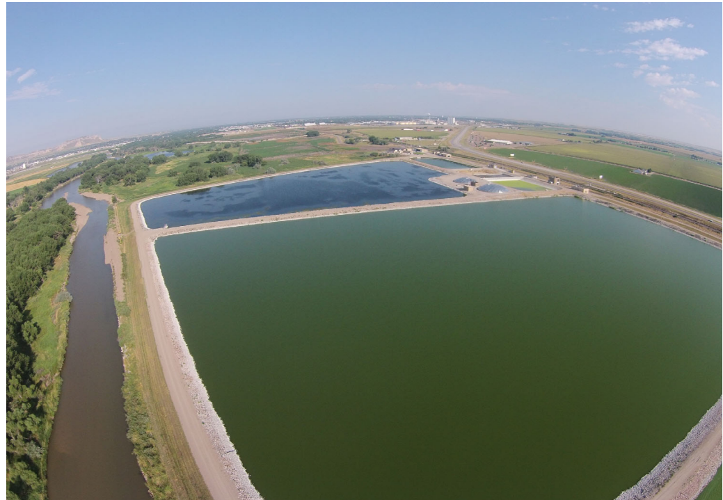
City of Scottsbluff, Wastewater Treatment Plant
