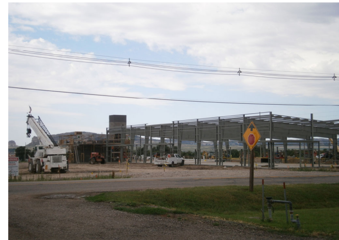
Elite Health Professional Medical Office Building 42nd Street & Avenue I
