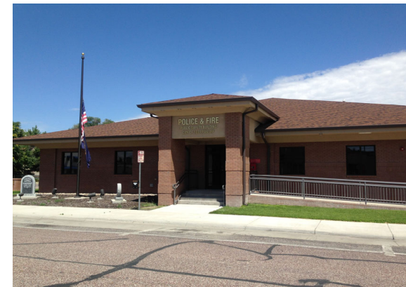
Public Safety Building - West 18th & Avenue B
