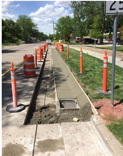
18th Street & 3rd Avenue
