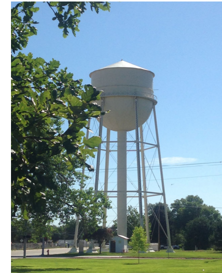
Water Tower - 27th Street & 2nd Avenue
