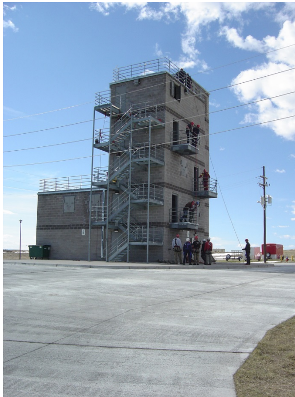
Example of a five-story tower with interior and exterior stairwells. The first and second floors have a larger footprint to mimic an apartment/office/hotel floor plan.
