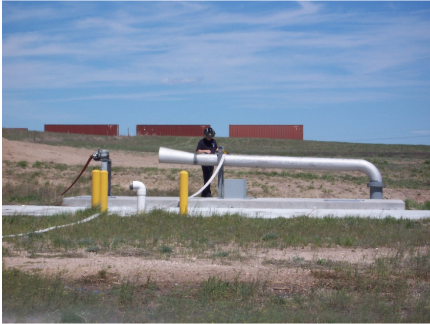
Example of a draft pit. The collection tube recycles the water to the holding tank below ground.
