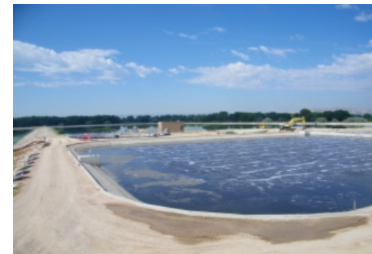
Aeration Basin - City of Scottsbluff Wastewater Treatment Plant
