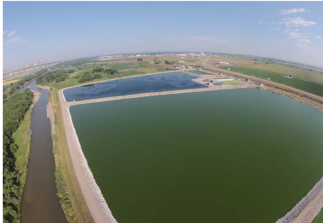
City of Scottsbluff, Wastewater Treatment Plant
