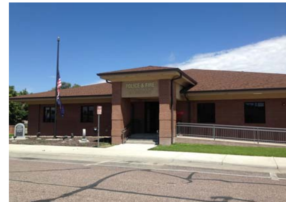
Public Safety Building - West 18th & Avenue B
