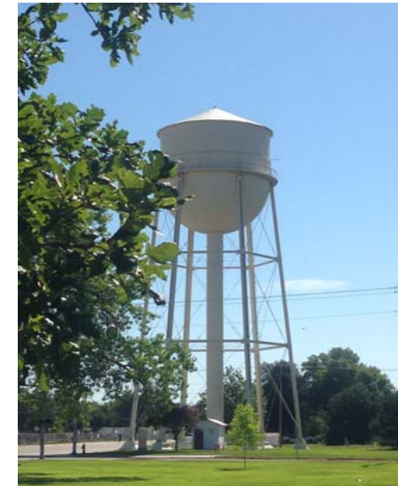
Water Tower - 27th Street & 2nd Avenue
