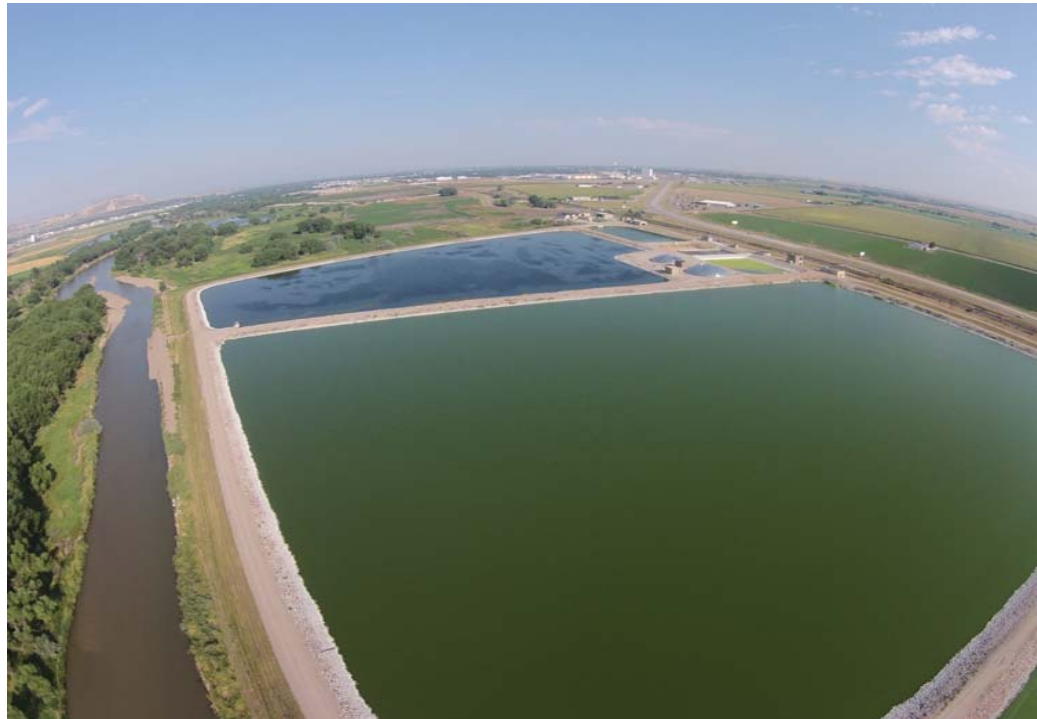
City of Scottsbluff, Wastewater Treatment Plant
