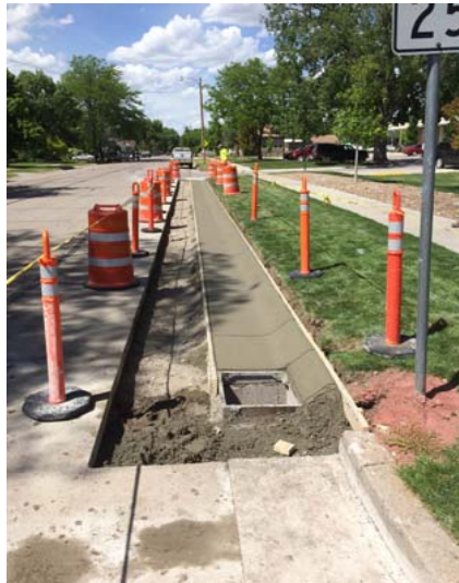
18th Street & 3rd Avenue
