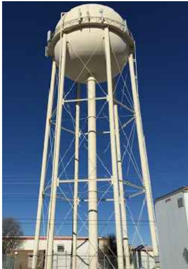
1 EXISTING TOWER PHOTO N.T.S.
