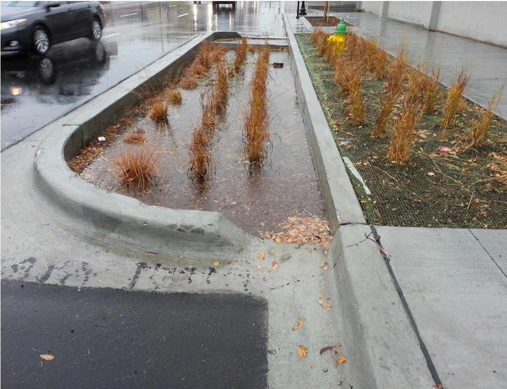
Example flow through urban raingarden
