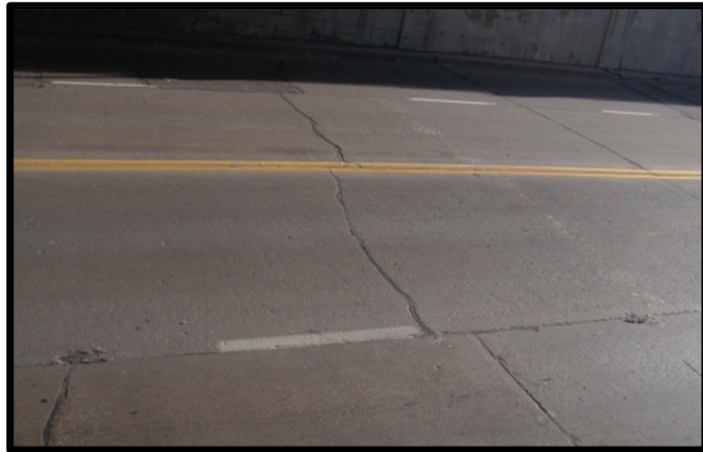
Photo 2.9: Typical Eddy Street Underpass transverse cracks.
