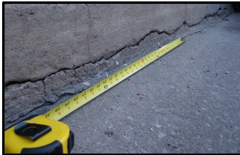
Photo 2.4: Typical horizontal crack.
