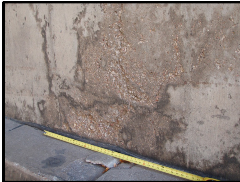
Photo 3.1: Typical spall.
