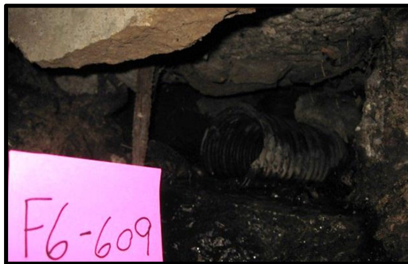
Photo 2.13: Eddy Street Underpass HDPE drain tiles outlet to Inlet F6-609.
