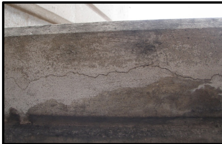
Photo 2.6: Mill Drive Bridge, random map cracking and minor spalls.
