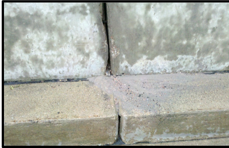
Photo 3.3 – Backfill migration.
