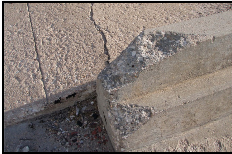
Photo 3.6: Industry Overpass Bridge, popouts and spalling.
