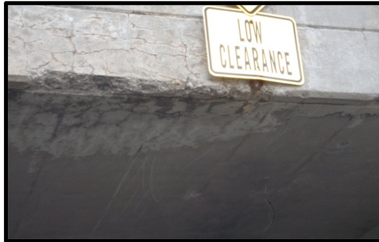
Photo 3.8: S. Front Street Bridge, severe cracking.
