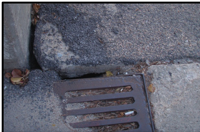
Photo 3.12: Sycamore Street Underpass walkway grate inlet, with voids under walkway.
