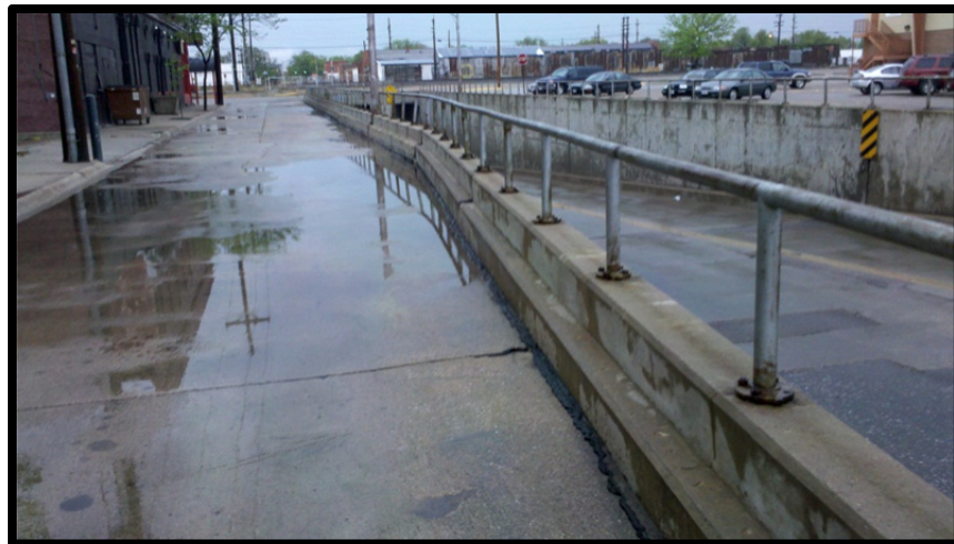
Photo 3.10: Sycamore Street Underpass, example of poorly draining pavement located adjacent to west retaining wall approximately 190 feet north of south end of the underpass. Ponded water infiltrates the pavement joints, resulting in soil migration through retaining wall joints.
