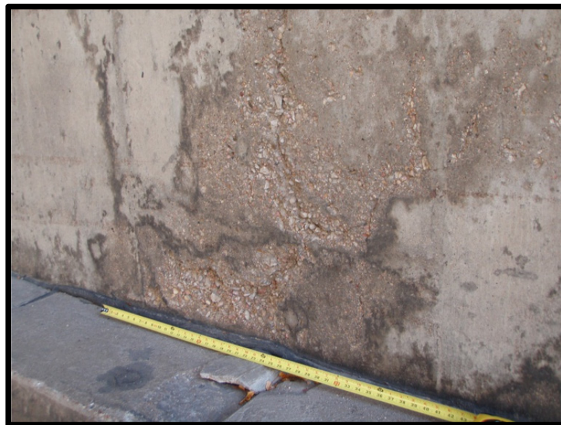
Photo 3.1: Typical spall.
