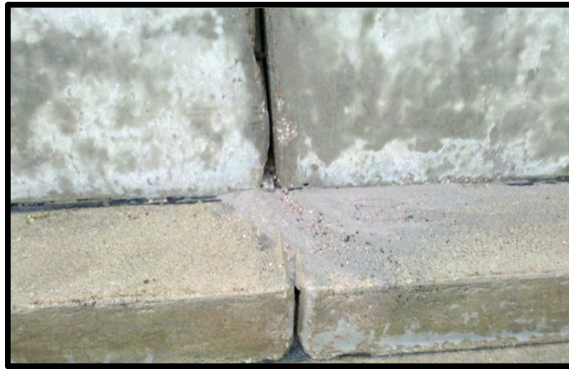
Photo 3.3 – Backfill migration.
