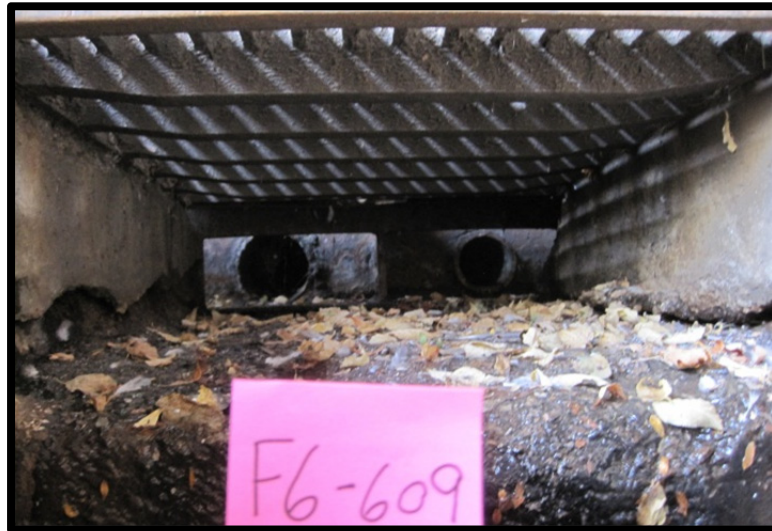
Photo 2.12: Eddy Street Underpass clay drain tiles outlet to Inlet F6-609.
