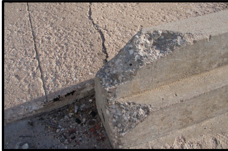
Photo 3.6: Industry Overpass Bridge, popouts and spalling.
