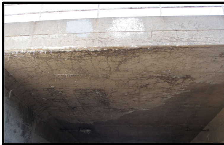
Photo 3.7: S. Front Street Bridge, severe cracking.
