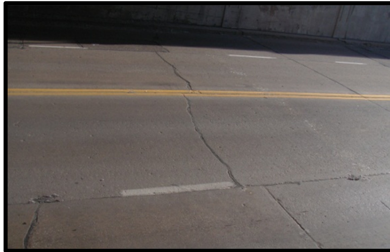
Photo 2.9: Typical Eddy Street Underpass transverse cracks.
