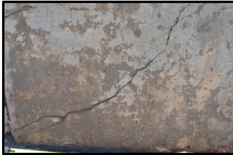
Photo 3.5: Horizontal crack.
