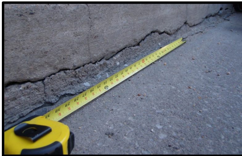
Photo 2.4: Typical horizontal crack.
