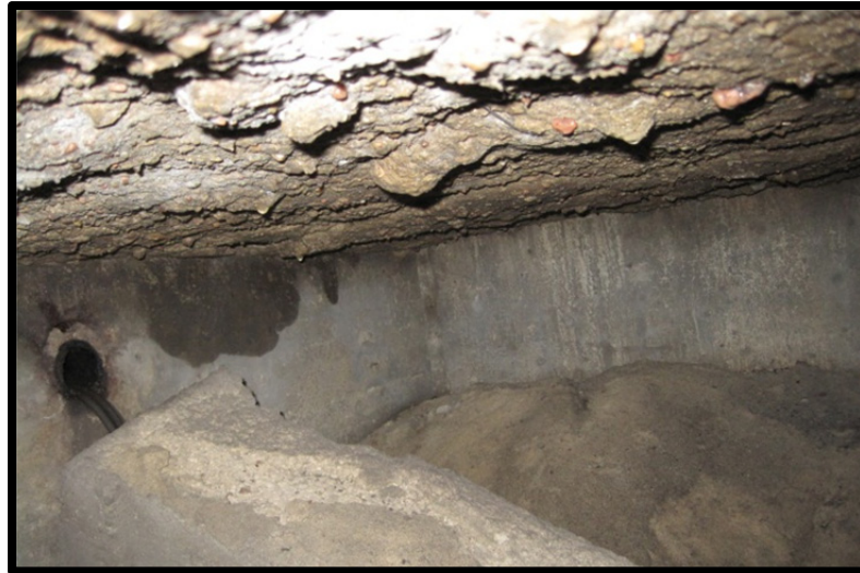
Photo 2.11: Eddy Street Underpass, loss of backfill material below walkway.
