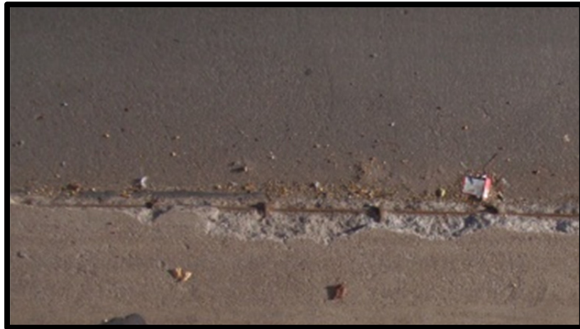
Photo 2.10: Typical Eddy Street Underpass curb spalling along west curb line.
