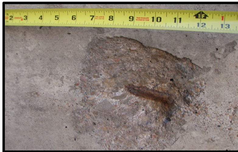
Photo 2.1: Typical spalls.
