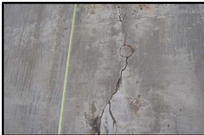
Photo 3.4: Vertical cracks.
