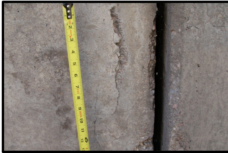
Photo 2.3: Typical vertical crack.
