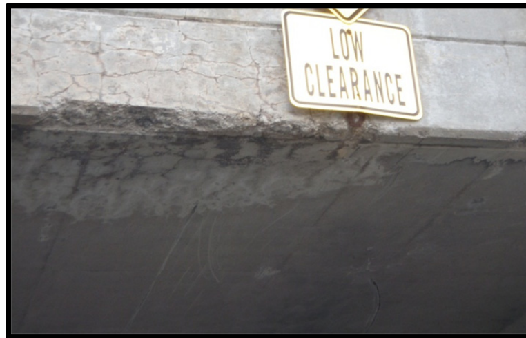
Photo 3.8: S. Front Street Bridge, severe cracking.
