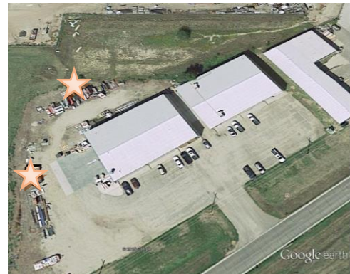
Unsecured materials Source: Google Earth August 2013 aerial
