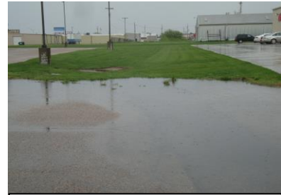
Standing water during a recent rain event
