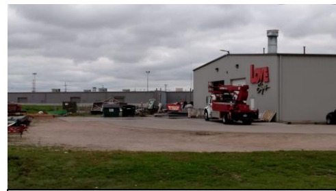
Photograph from Old US Highway 30 Source: Marvin Planning Consultants
