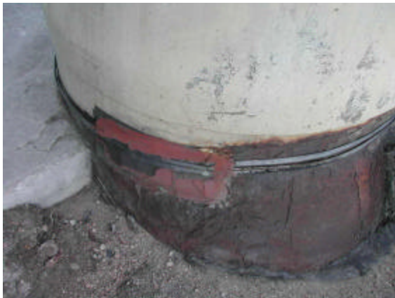
Figure 3 East Riser Patch
