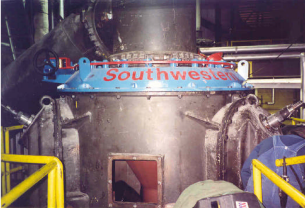
Installed Pulverizer Separator Top and Classifier Assembly
