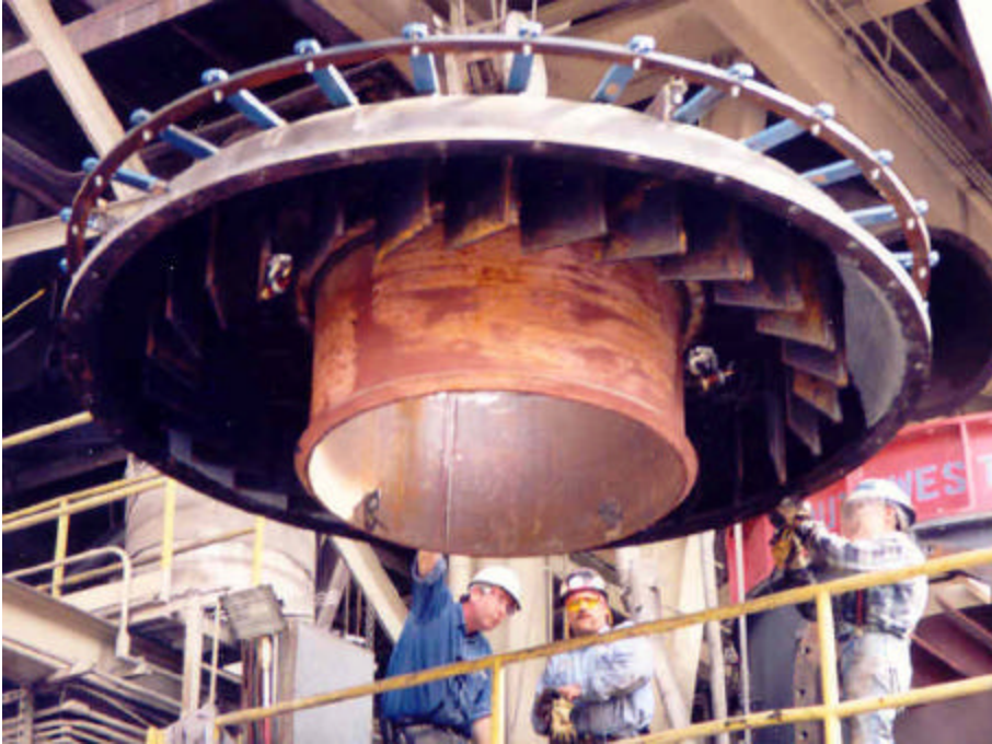
Pulverizer Separator Top and Classifier Assembly
