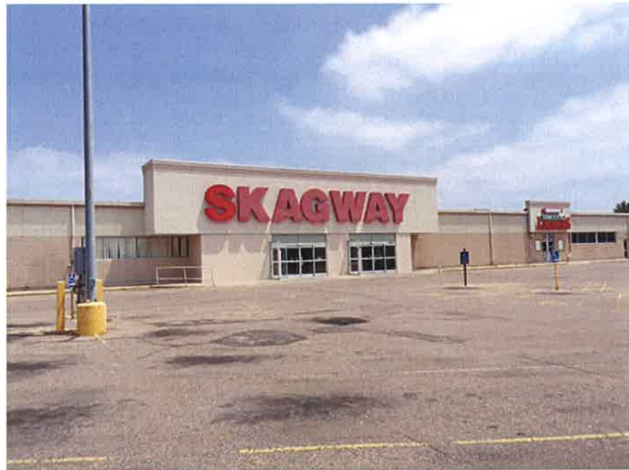
West Front Facade
