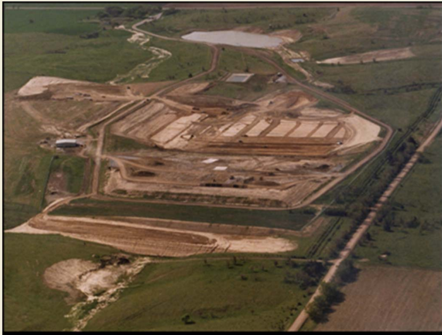
Landfill on Husker Hwy @ Hall / Buffalo County Line
