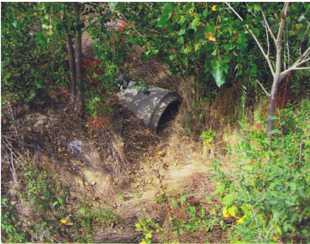
Strom sewer outlet. Hole dug out around pipe. About 100' west of Cherokee Ave.
