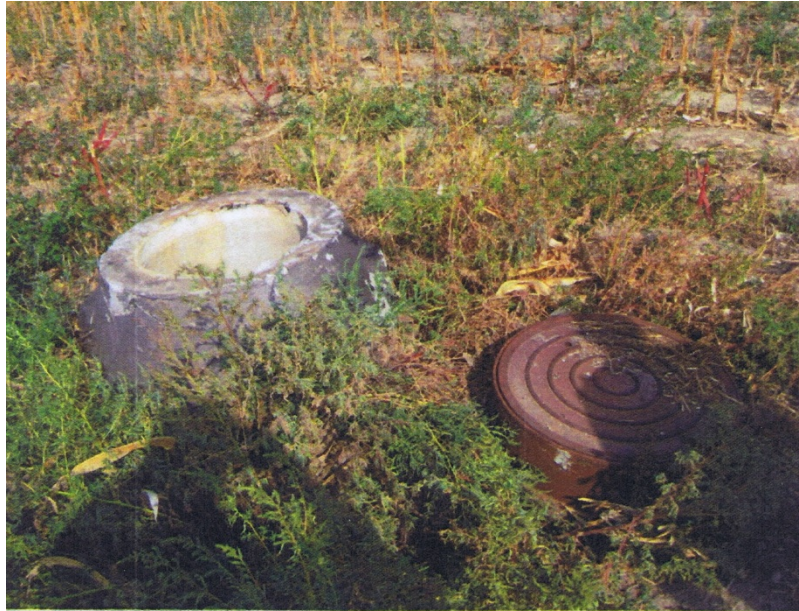
Sanitary sewer manhole.
