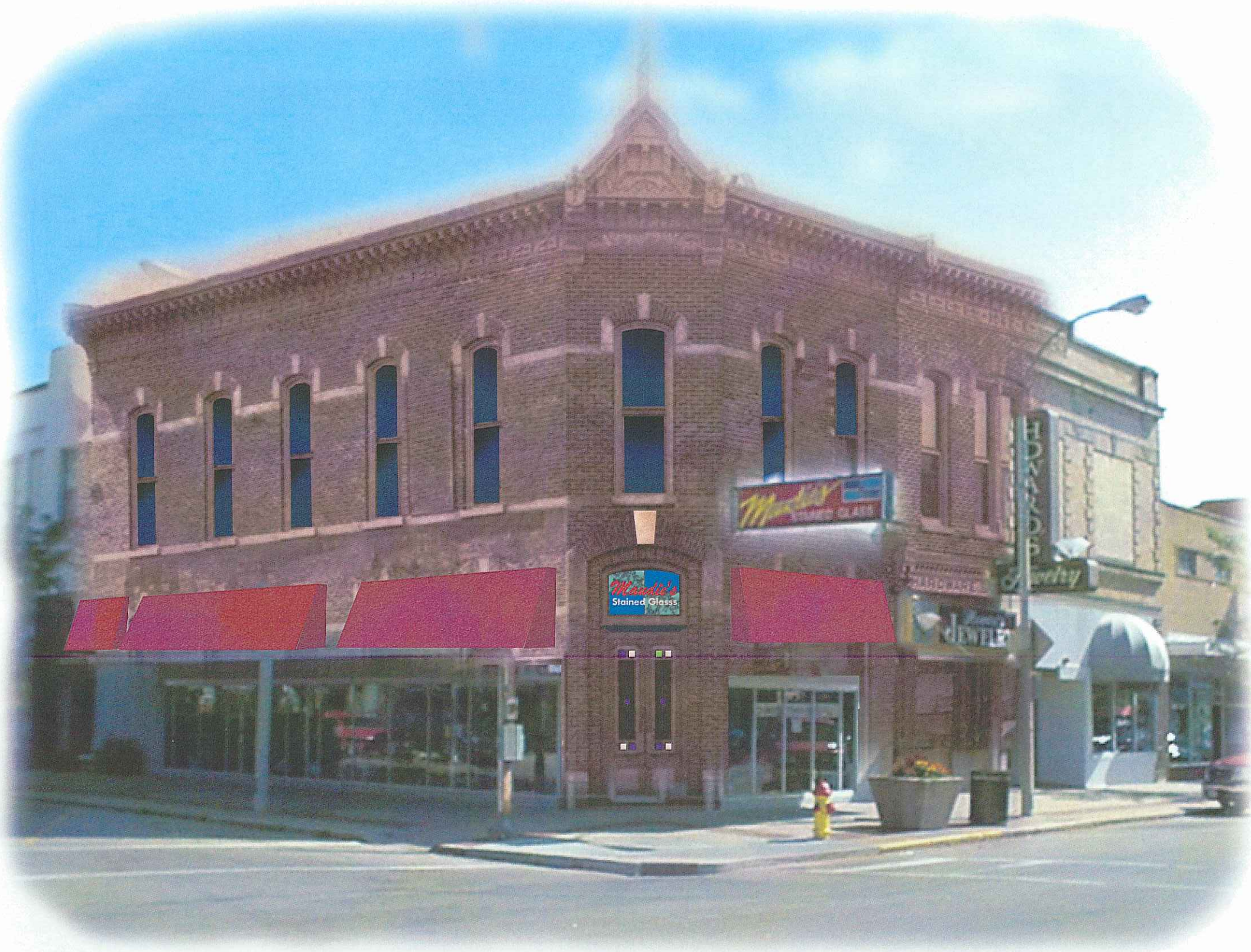
THE RESTORATION GOAL IS TO REPLACE MUCH OF THE ARCHITECTURE ACCORDING TO THE ORIGINAL BUILDING STYLE INCLUDING THE BRICK COLOR, PEDIMENT AND CORNICE SHAPES AND WINDOW TREATMENT.
