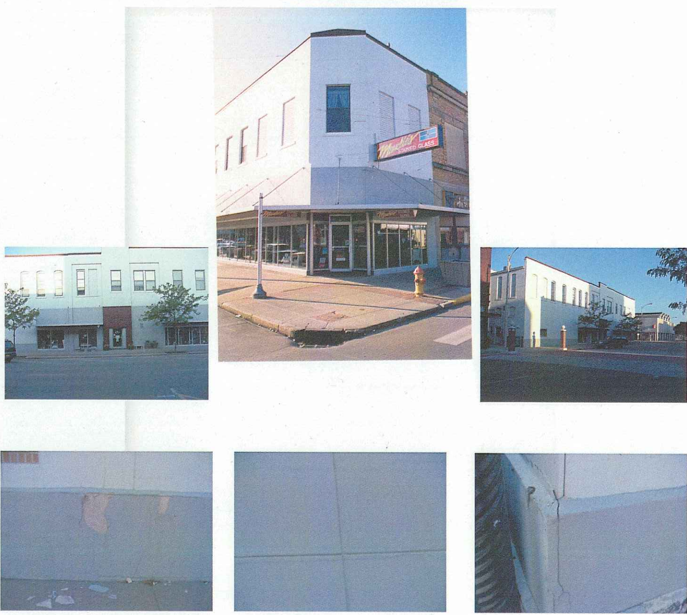
THE STUCCO IS RAPIDLY FAILING AND IS LEAKING ON THE EAST AND NORTH SIDES OF THE BUILDING.
