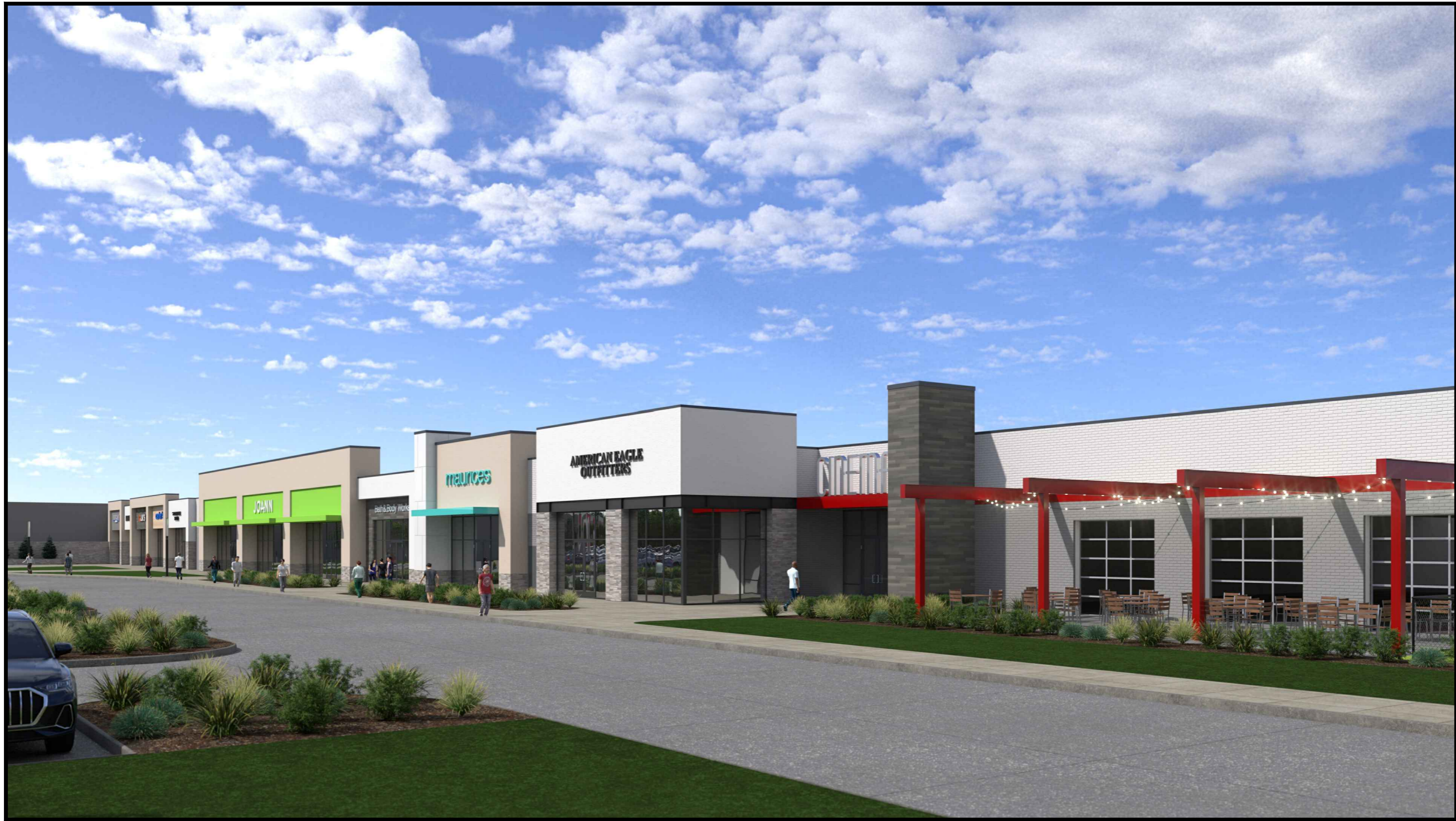
Eastern Facing Storefronts Towards Webb Road
