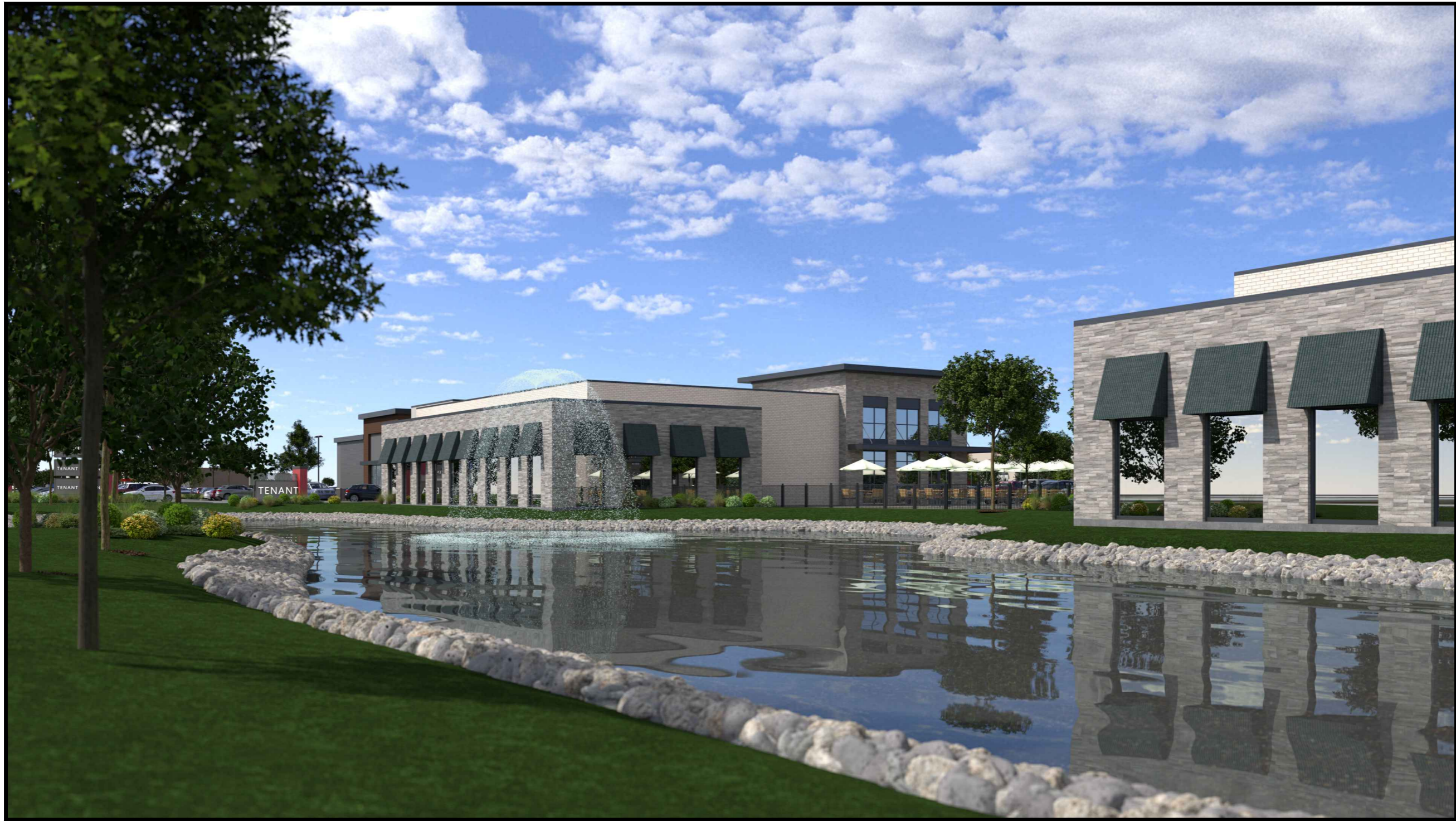
Future Sit-Down Restaurants Looking East from Highway 281
