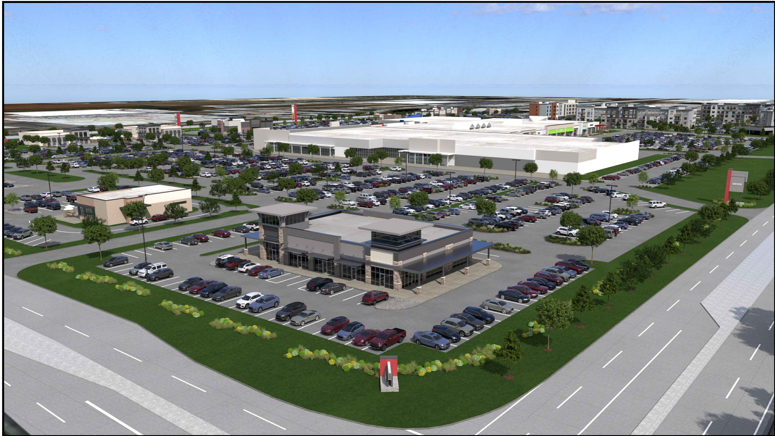
Looking Northwest From Corner of 13th Street
