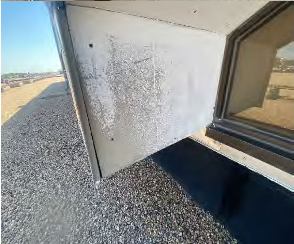
Photo 14: View of Assumed transite soffit.
