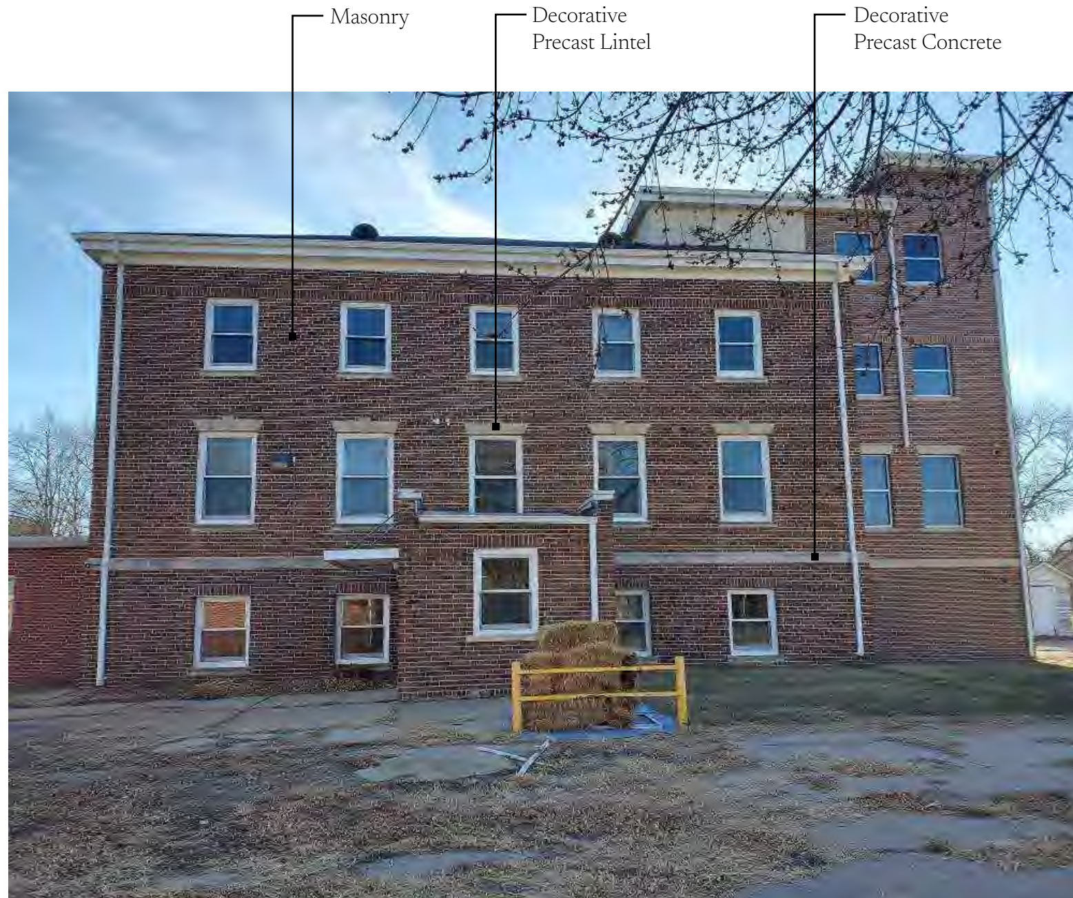
*Material notation notes existing materials. All existing facade materials and elements to remain unless noted otherwise.
