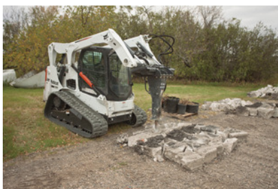
Example of Skid Steer/Compact Track Loader
