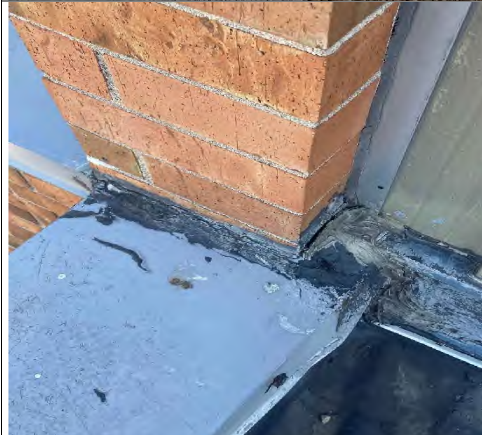
Photo 12: View of Sample SRR-2, material appears to be a patch material.
