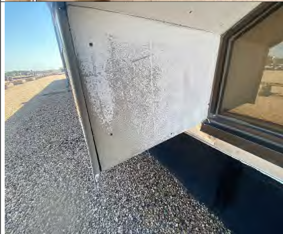
Photo 14: View of Assumed transite soffit.
