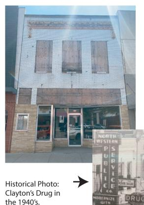
Replacement of old broken windows on second floor that have been covered for 50+ years Replacement of new brick front. Old brick is severely damaged Replacement of damaged windows and storefront entryway to allow for additional weather coverage Restructure landing of entryway
