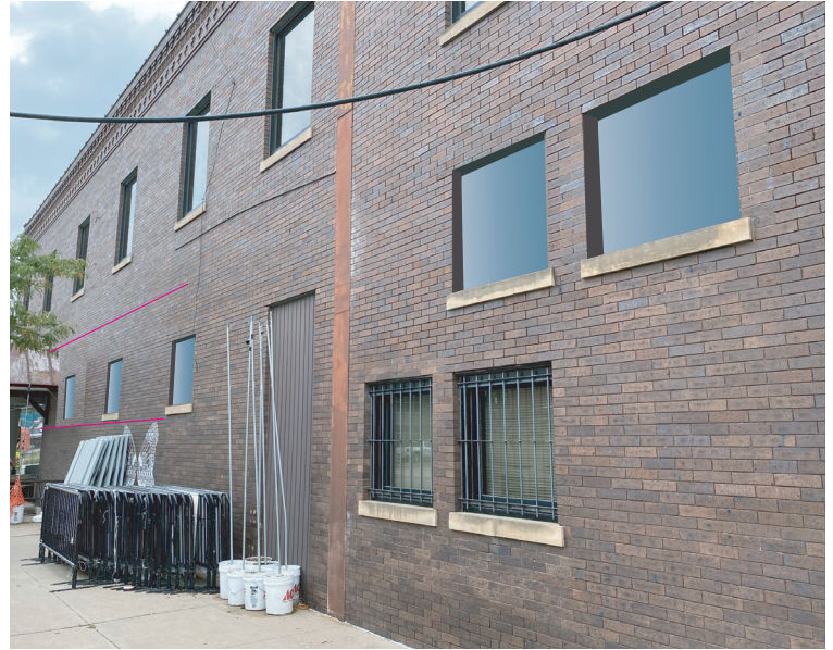
223 W 3rd Building Facade Proposed Bricked up Window Replacement - West side 1st Floor
