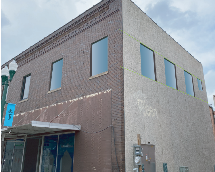
223 W 3rd Building Facade Proposed Bricked up Window Replacement - Southwest corner 2nd Floor
