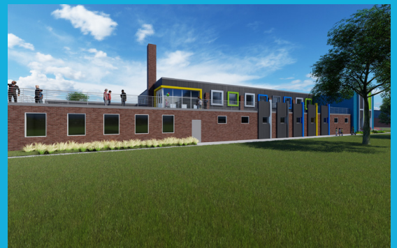
Rooftop access with gathering areas
