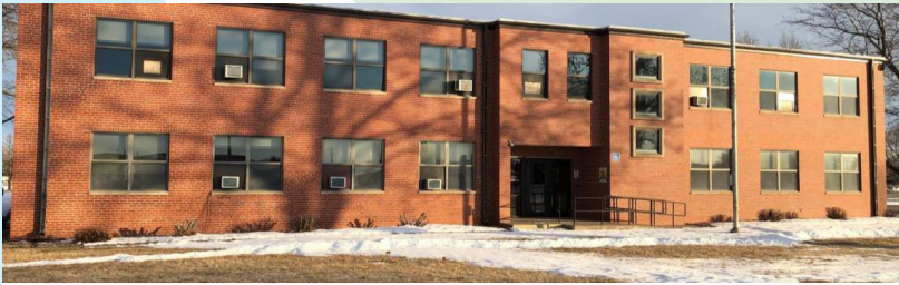
Existing former Armory Building located on Old Potash Hwy by Ryder Park
