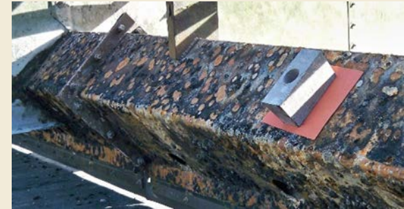
Anodes inhibit corrosion
