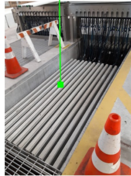
UV BULB CLEANING SYSTEM
