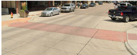
Curb Extensions, 3rd and Wheeler. Source: Google StreetView
