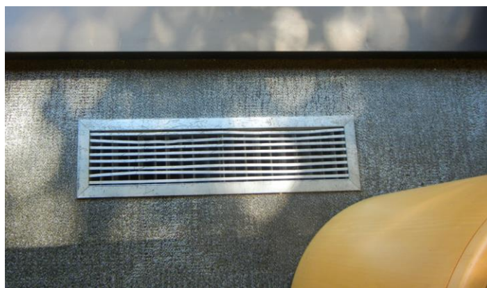
Floor Diffuser Example
