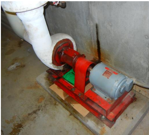
Hydronic Pump and Piping
