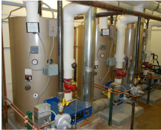
LES Fire Tube Boiler
