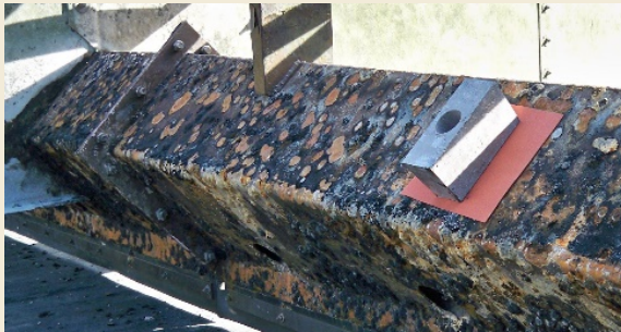
Anodes inhibit corrosion
