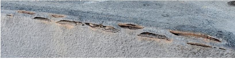
Rust/separation of frame
