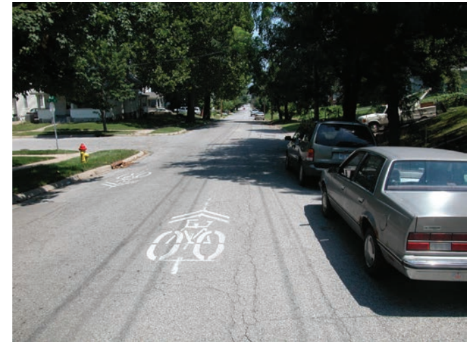
Marked routes. Left: Typical shared lane marking for a Grand Island street; Above: Shared lane marking installed.
