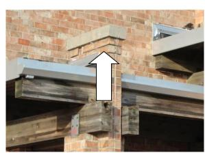
The exterior portion of the mall is beginning to show considerable wear, likely to deferred maintenance. In the photos above there are examples of where masonry construction has been compromised and is in danger of falling from the building onto the ground. Base upon a visual ground inspection, it appears like there is considerable water penetration in the brick and mortar system.
