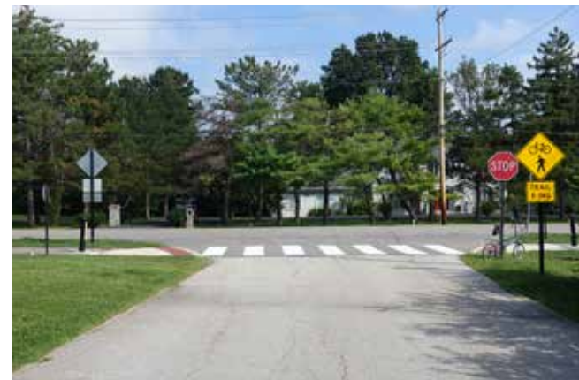
Top: Capital Avenue Trail. Above: Clayton Road sidepath in St. Louis County, Missouri. Note the highly visible crosswalk using high visibility markings and use of the trail crossing stack sign on intersecting streets.
